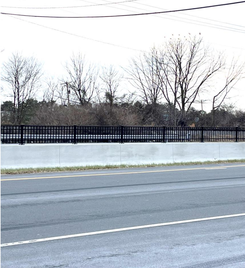
Barrier with Fence (Locations with Narrow Median)
